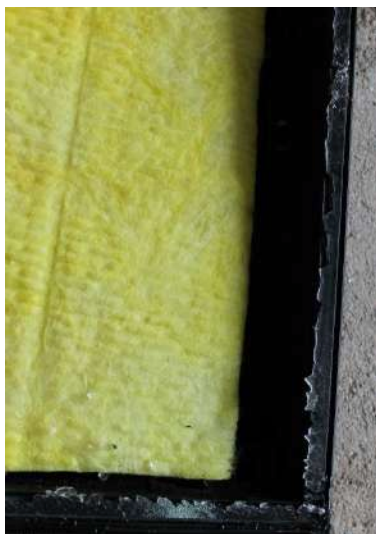
Fig. 6: final inspection 终检
